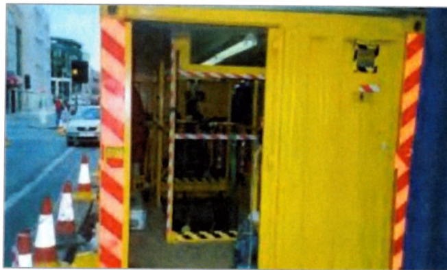
Figure 9 - HV cable jointing container
