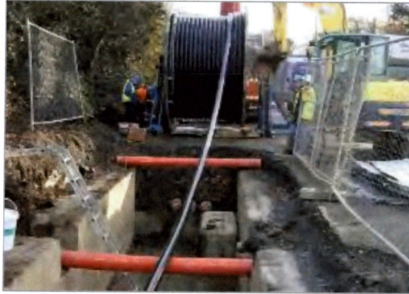
Figure 8 - HV cable pulling procedure (Typical drum set-up)
