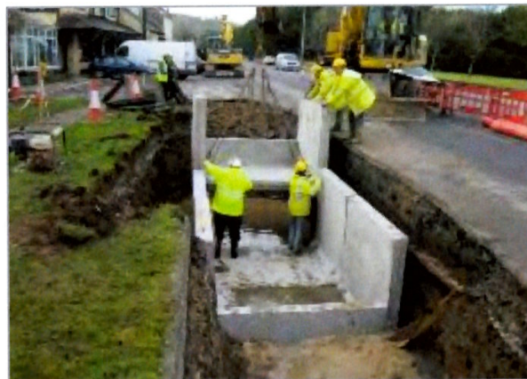
Figure 7 - Typical joint bay under construction (pre-cast)
