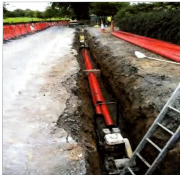
Figure 2 - Typical 110kV Underground Duct Installation
